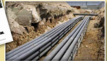
Utility Corridor Modernization
