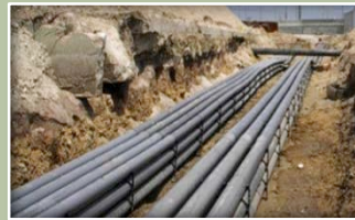
Utility Corridor Modernization
